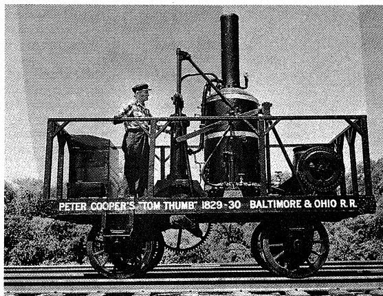
The Tom Thumb , first American-built locomotive to operate in regular service
